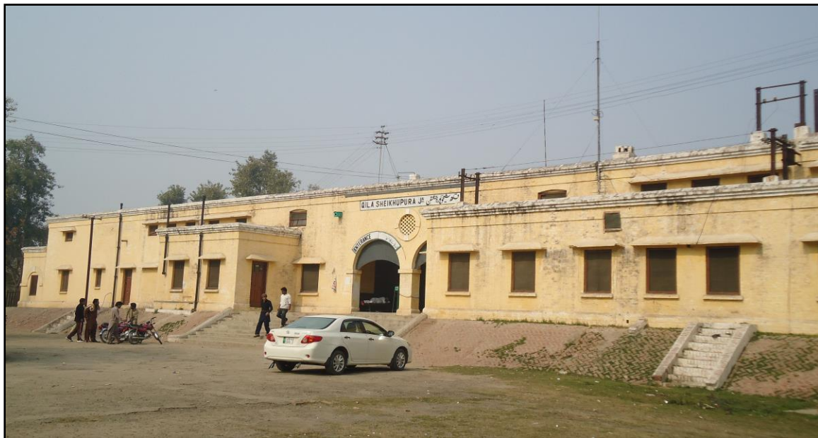
Figure 18: Railway Station, Sheikhupura (Photograph by the Principal Author).
