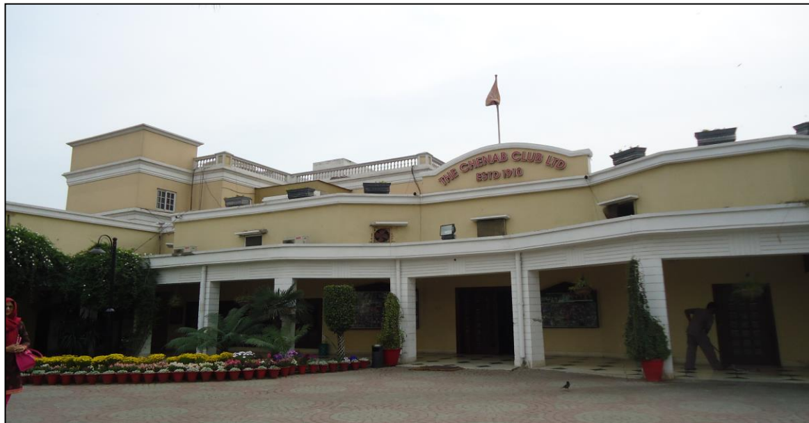
Figure 25: Chenab Club, Lyallpur, built in 1910 (Photograph by the Principal Author)
