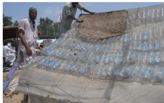
Figure.7. Tent-I under construction
