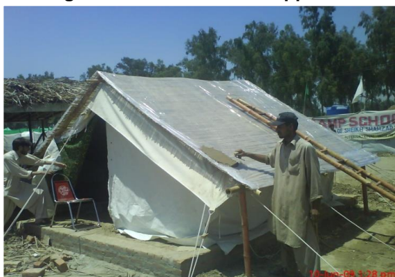
Figure.8: Tent-02 During construction Stage
